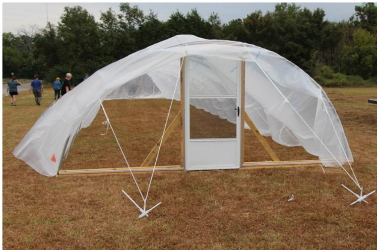
The training covered the **latest refinements** that have emerged from the work the Kerr Center has done using the design over the past few years, including both a **more secure anchor design**, and an **improved approach to endwall construction and attachment**. Workshop participants received a printed set of **plans and instructions for building a hoop house of this design**, streamlined to just 8 pages, and including a materials list and estimated costs.
