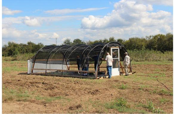
The pipe frame isn't nearly as large as the full hoop house design - only 14' x 23', as opposed to 17' x 100'. However, it is rigid, and the bottom members of the pipe frame can act as skids, making the **entire structure portable.**
