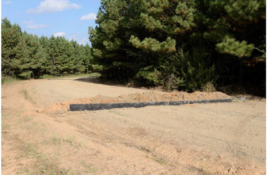
Some of the ranch roads are serving as **experimental areas** for the addition of "water bars." These consist of used mining belts buried in the actual roadbed at an angle of 30-40 degrees, with the goal of [reducing erosion](#). The performance of these initial installations will be monitored, and they can be expanded if they prove effective.
