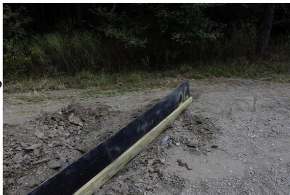
The conveyor belt should be set with at least a 30% angle to the road, and should only leave 4-5 inches exposed above the road surface, so that a vehicle can cross it. The conveyor belt diverters are not for roads with heavy traffic.
